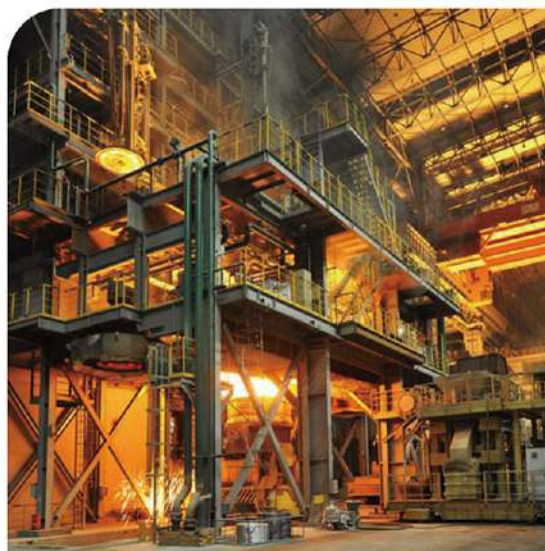
RH 精炼炉 RH REFINING FURNACE
